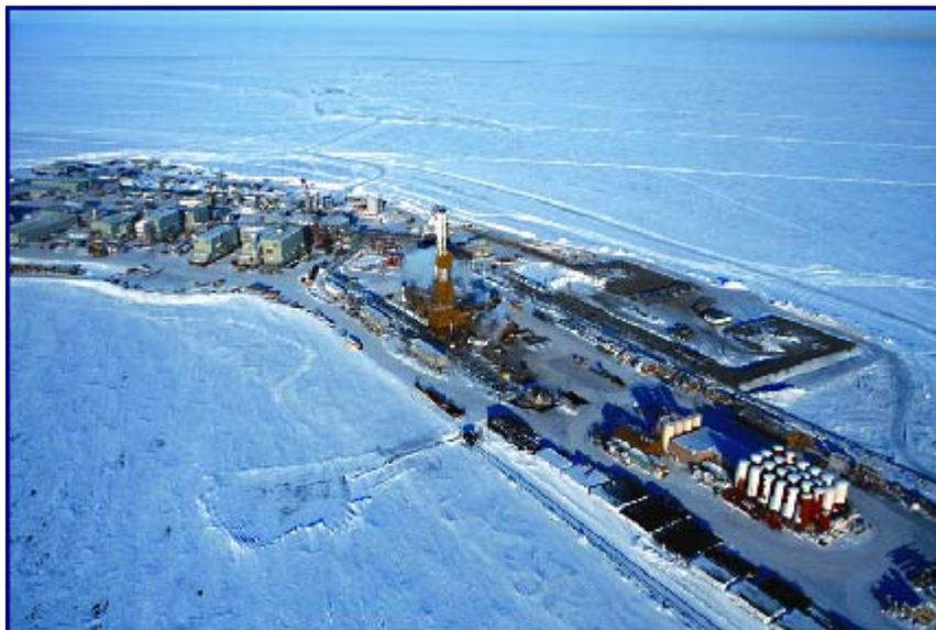
In Alaska, improved technology, closer well spacing and directional drilling have enabled 40-thousand-acre fields like Alpine on Alaska's North Slope, to be developed with less than 100 acres of surface disturbance.
