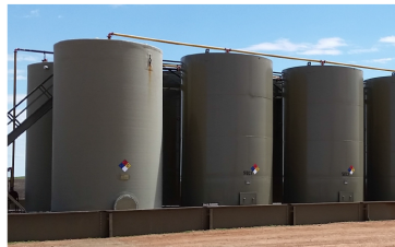
Storage vessels at an oil and gas production facility.
