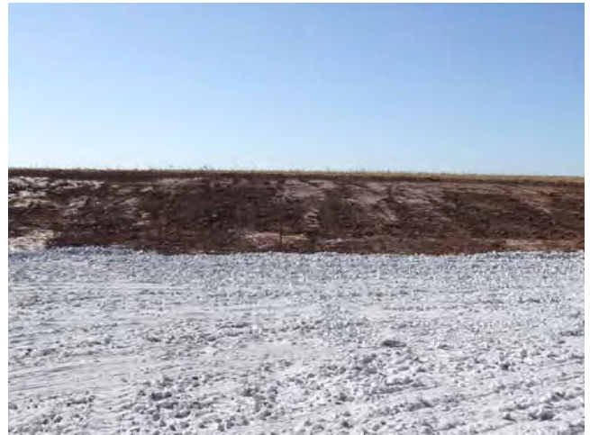
Cut Side Stabilization
