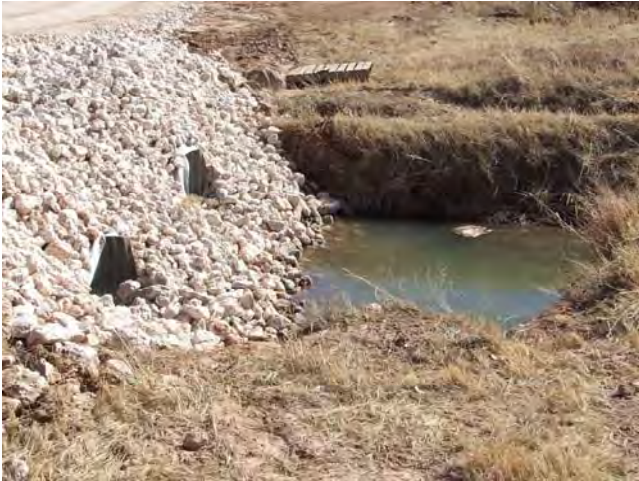
Surge Road & Culvert Installation
