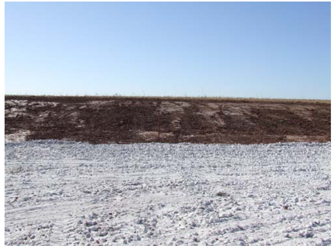
Cut Side Stabilization
