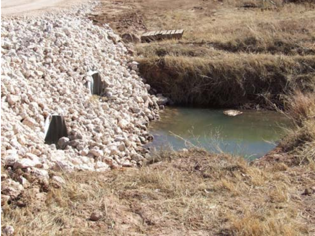
Surge Road & Culvert Installation
